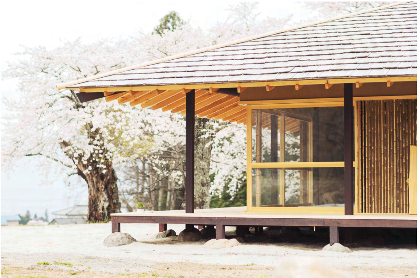
Sobokuya's office with “Ishibadate” stone base
