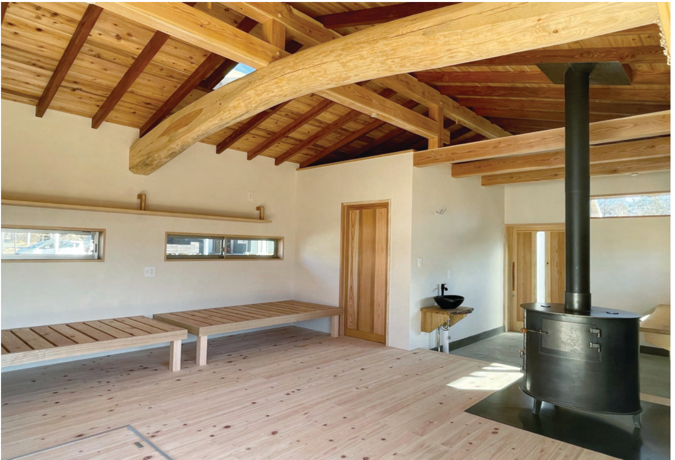
A natural “Taiko beam” in the middle of the house
